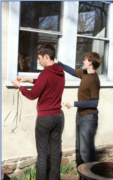
Window tape patterns are easy to apply and provide an effective deterrent against bird strikes.
