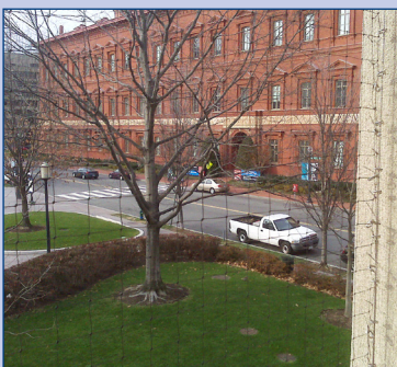
Window netting provides a see-through screen that will cut down on bird strikes. Photo: John Pace, BirdMaster Bird Control Systems
